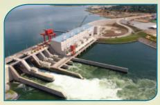
concrete gravity dam. It has a concrete powerhouse structure, with an integral intake, five double-regulated Kaplan turbines, and a 132 kV substation.
