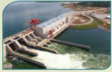
powerhouse structure, with an integral intake, five double-regulated Kaplan turbines, and a 132 kV substation.
