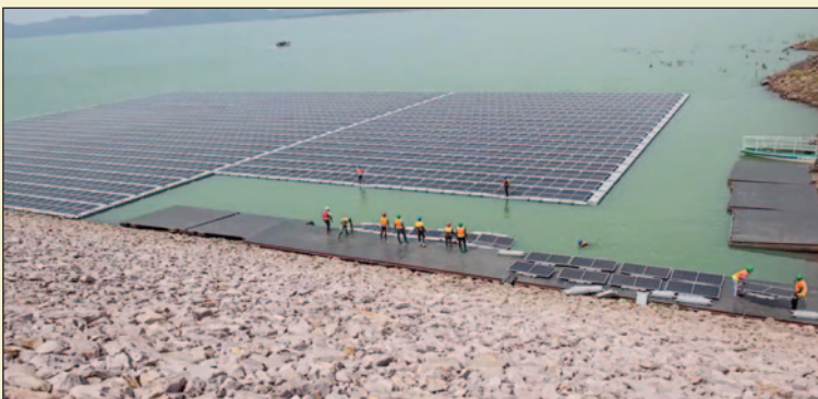
The 1 MW pilot FPV project, on the Bui reservoir in Ghana, described by Anthony Osafo-Kissi of the Bui Power Authority.
