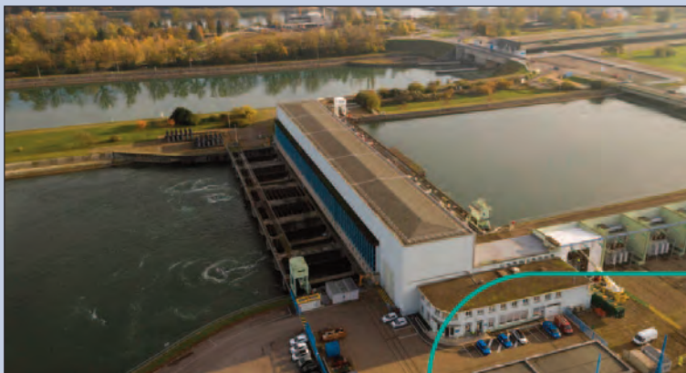
The Vogelgrün plant in eastern France, one of the XFLEX demonstrator projects. Jean-Louis Drommi of EDF explained that as part of the XFLEX project, one of the Kaplan units at the plant will be hybridized with a small battery; both will work in tandem under the control of a specific power sharing algorithm.
