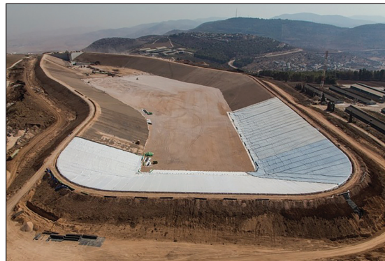
Mount Gilboa pumped-storage project under construction in Israel. Source: Admir Technologies.
